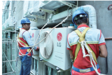
Air conditioner maintenance service
