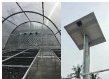
Solar dryers for drying agriculture products & salt
